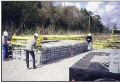
Each mat is loaded onto the truck by a spreader bar attached by six connections on each end.
