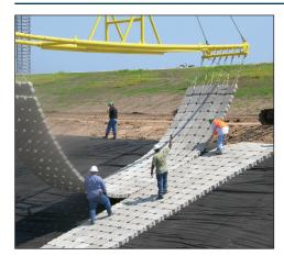
SHOREBLOCK® BD mattresses are pre-assembled to the size specified for the project. Fabrication of a SHOREBLOCK® BD mat is accomplished by threading polyester cable in both directions through a series of blocks.
